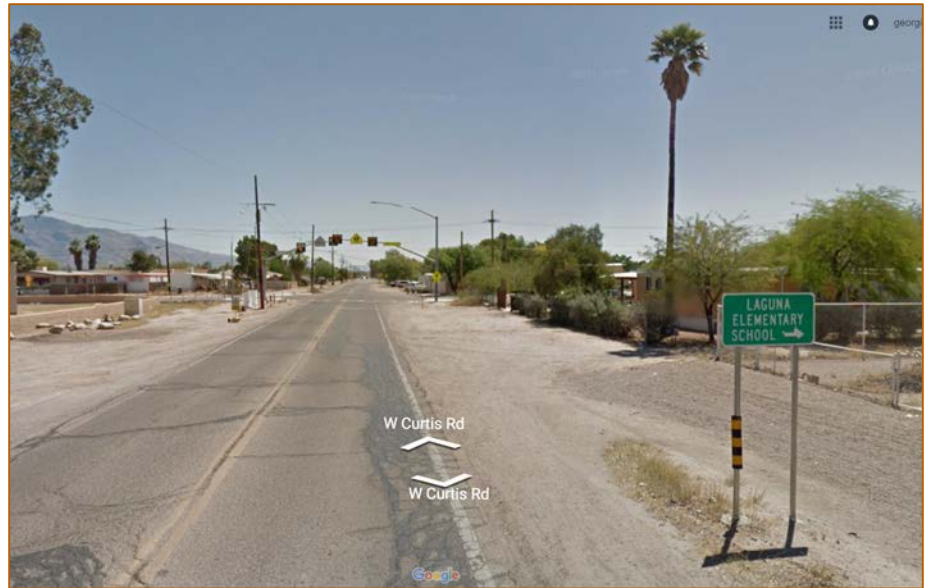
Figure 17. Wayfinding signage does not offer safety message.
