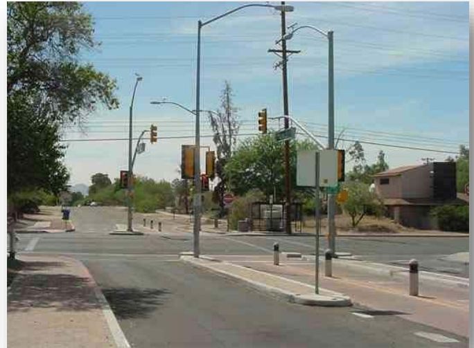
Figure 33: Example of a TOUCAN signal in Tucson
