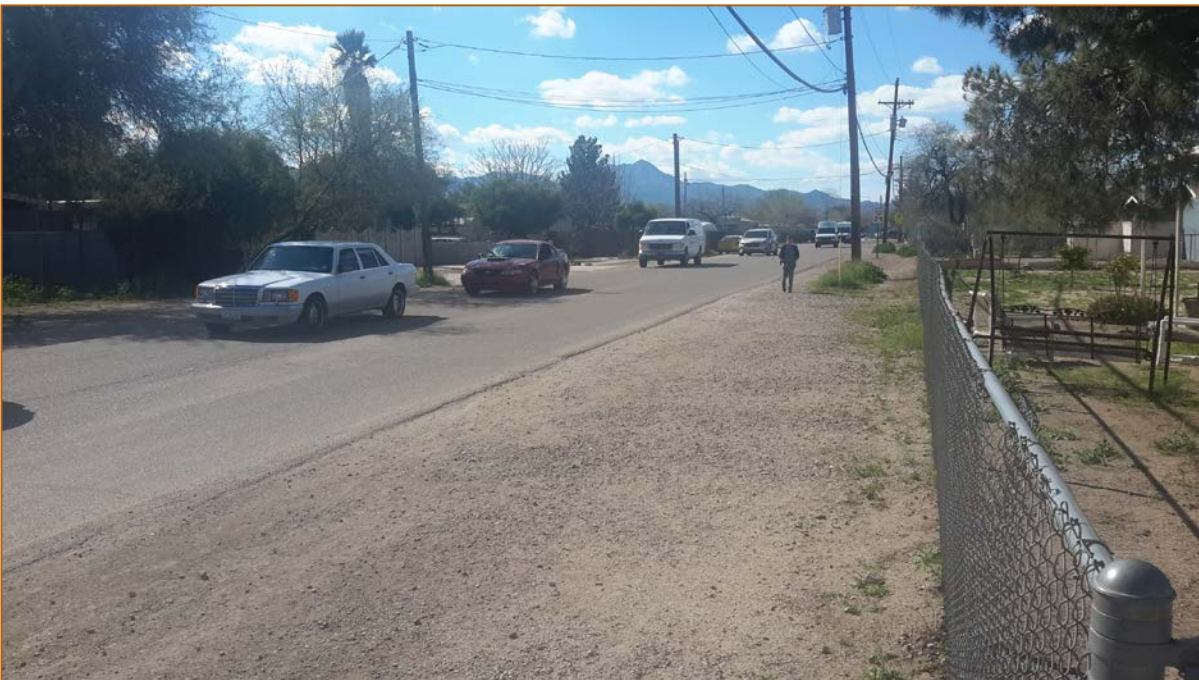
Figure 11: Pedestrians traveling along W. Diamond Street must use the dirt and gravel shoulder.
