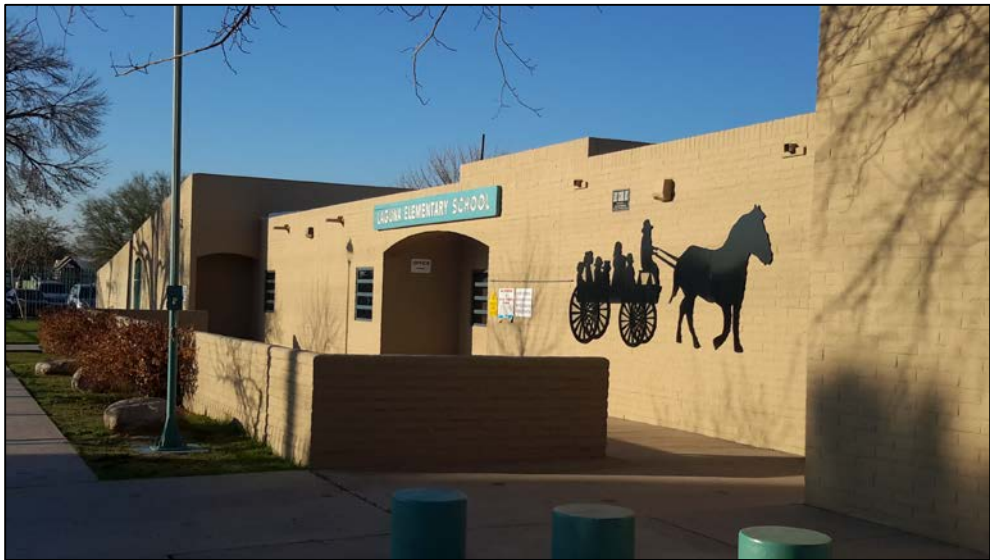
Figure 6. Laguna Elementary School main entrance on N. Shannon Road.
