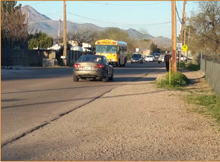
Figure 16. Faded edge lines diminish the separation between the roadway and shoulder.
